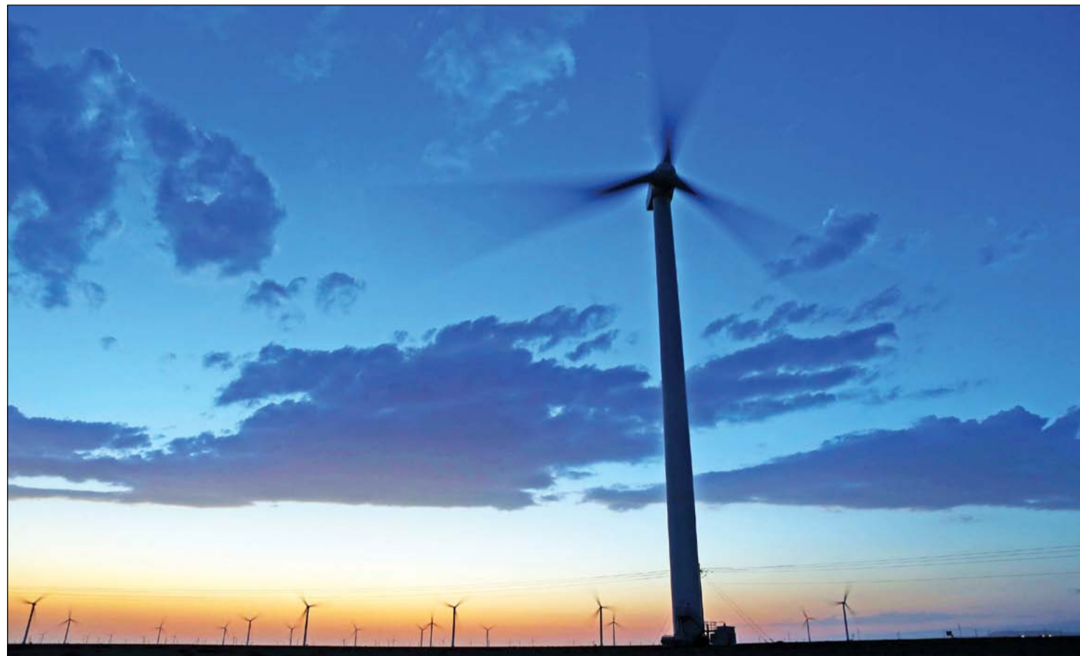
A wind turbine system generates energy in Northwest China's Xinjiang Uygur autonomous region. China has made a huge investment in wind and solar power to promote green development as President Xi Jinping calls for an end to environmentally damaging practices. XINHUA
